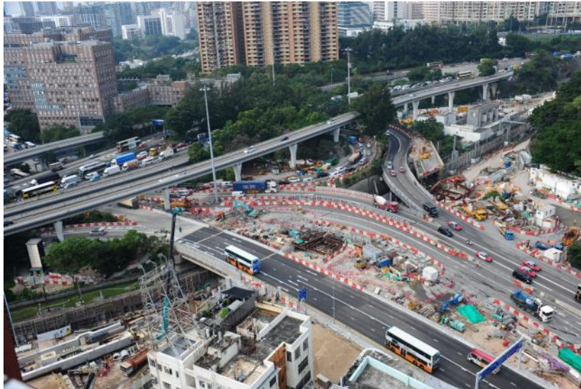
Tunnel excavation under Chatham Road North and near Winslow Street
