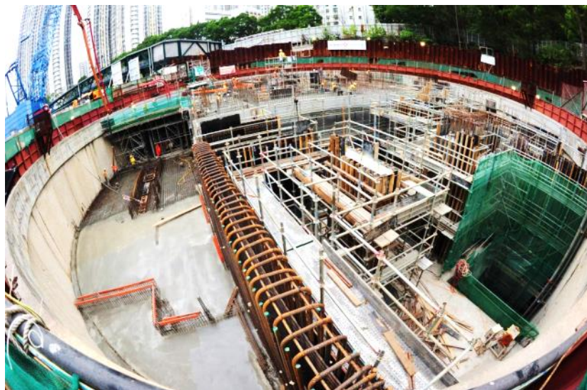
Structural works for the ventilation building at Ma Chai Hang
