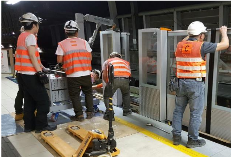
Retrofitting works of APGs
