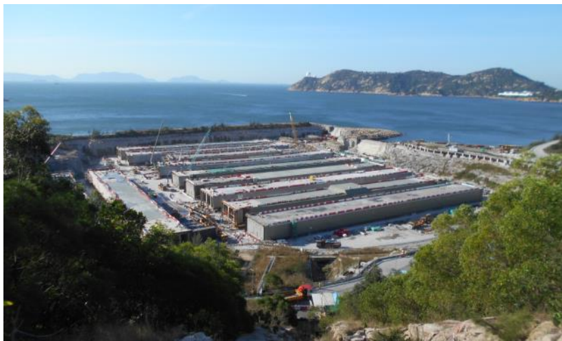
Structural works of IMT pre-cast units are substantially completed
