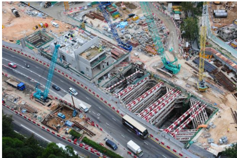
Expansion works for Diamond Hill Station
