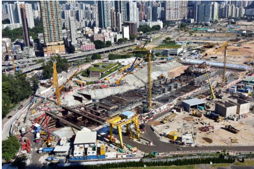
Structural works for To Kwa Wan Station
