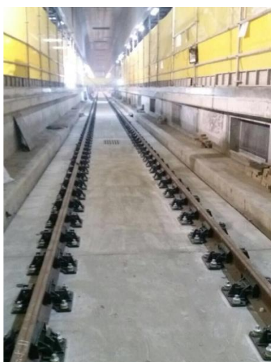
Completion of track-laying works at WKT platform level
