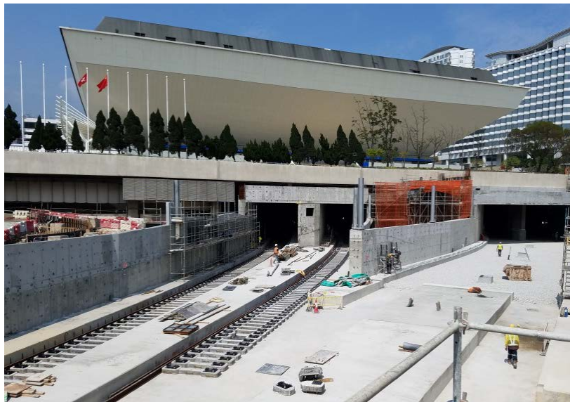
Track-laying works at Hung Hom stabling sidings
