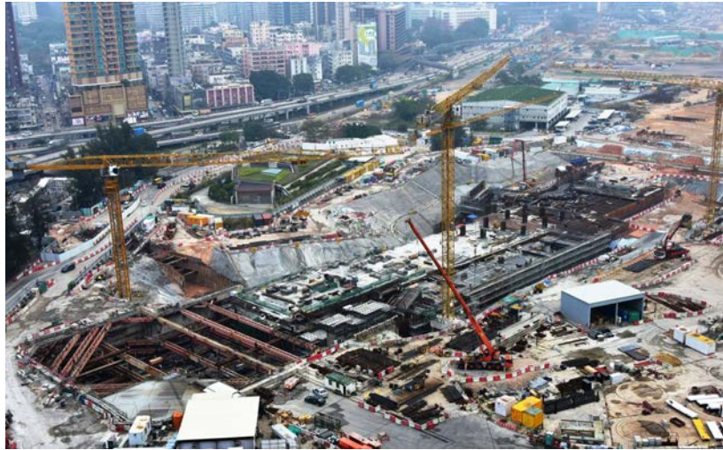
Structural works for To Kwa Wan Station
