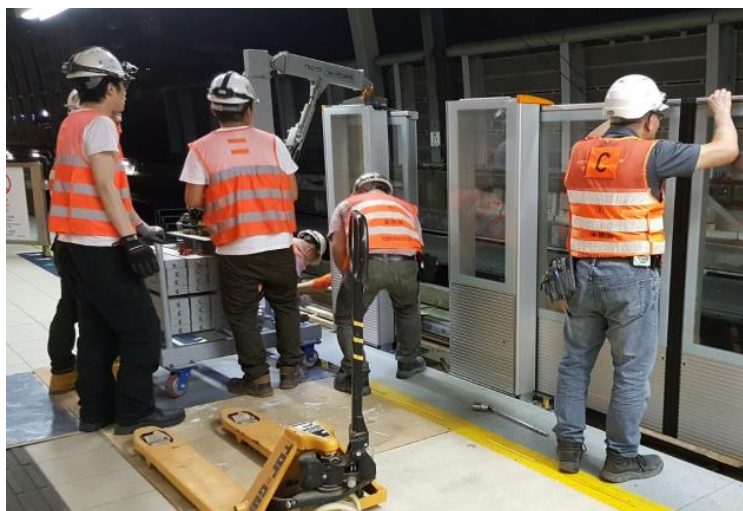
Retrofitting works of APGs
