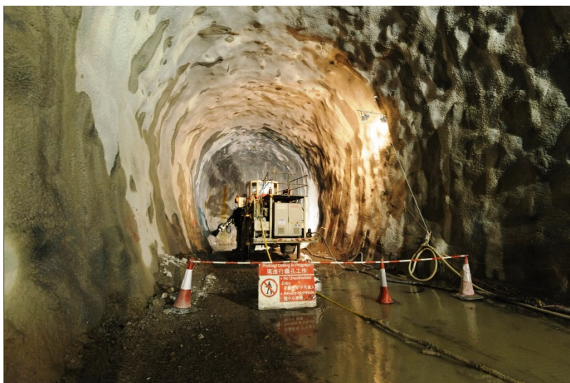
SCL overrun tunnel is being constructed by drill and blast method
