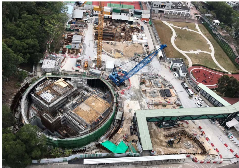
Structural works for the ventilation building at Ma Chai Hang
