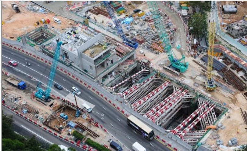
Expansion works for Diamond Hill Station
