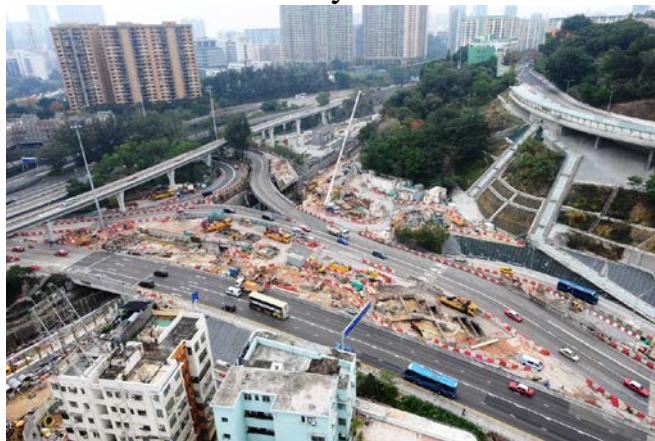
Structural works under Chatham Road North and near Winslow Street
