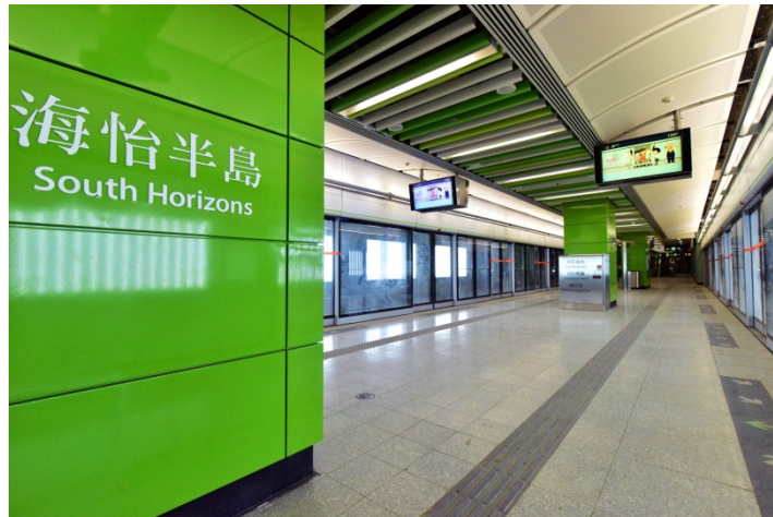
Construction is complete at South Horizons Station
