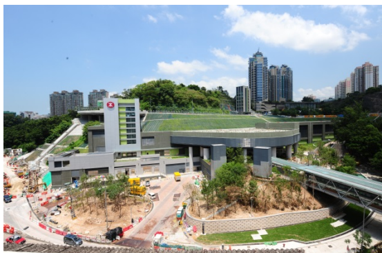
External finishing works of Ho Man Tin Station has been completed.
