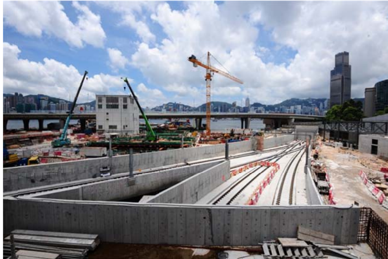
Track-laying works at Hung Hom stabling sidings
