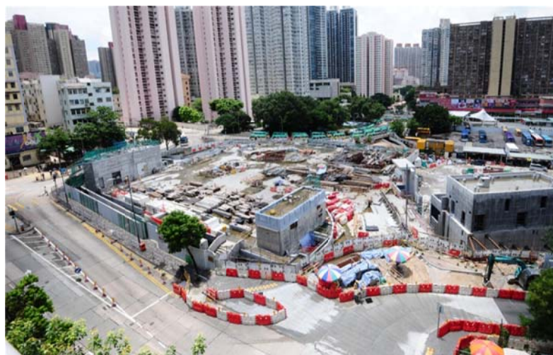
Emergency Access Point at Fung Tak
