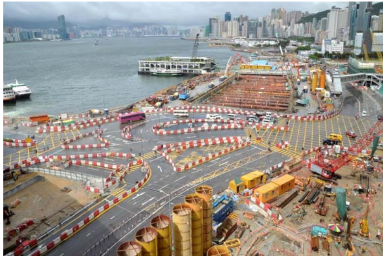
The junction between Convention Avenue, Fleming Road and Expo Drive East shifted eastward in phases
