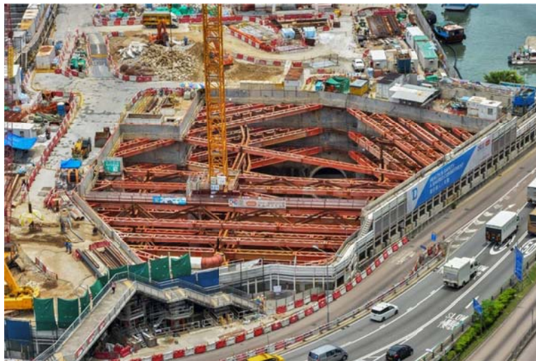
Excavation of the ventilation facilities at the former Police Officers' Club works site
