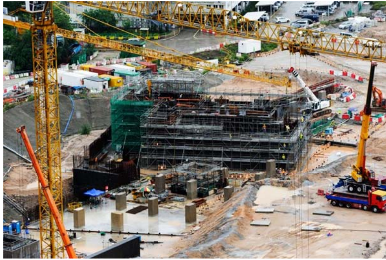
Structural works for To Kwa Wan Station
