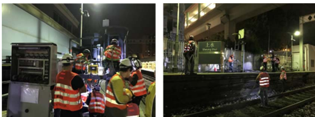
Signalling upgrade along EAL
