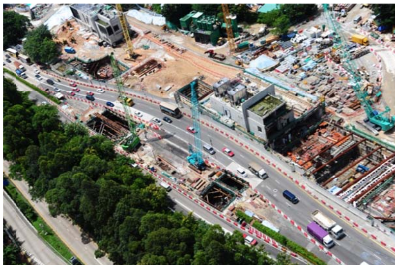
Expansion works for Diamond Hill Station
