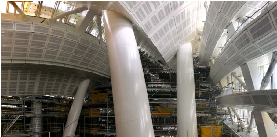
Installation of cladding panels inside the West Kowloon Station
