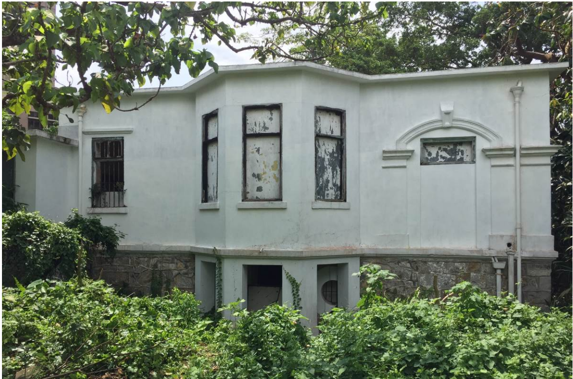
Existing Condition of the Old Dairy Farm Senior Staff Quarters 舊牛奶公司高級職員宿舍的現貌
