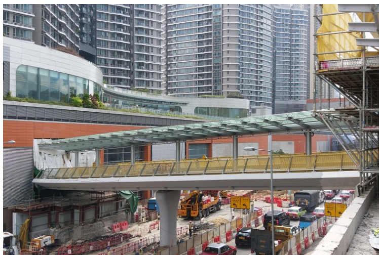
The footbridge connecting West Kowloon Station with Austin Station
