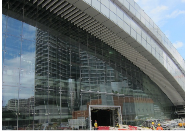
Construction of the eastern arch of the Station Entrance Building
