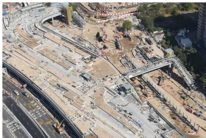
The West Kowloon Station Bus Terminus is being constructed
