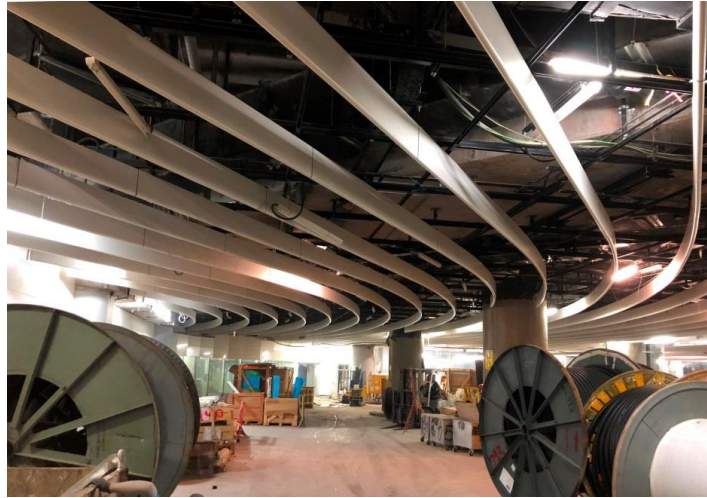
Taxi drop-off area at Level B1 of the West Kowloon Station
