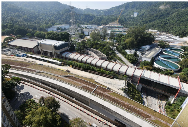
Viaduct and at-grade tunnel box
