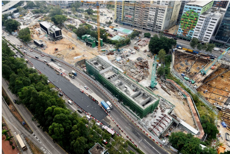
Expansion works for Diamond Hill Station
