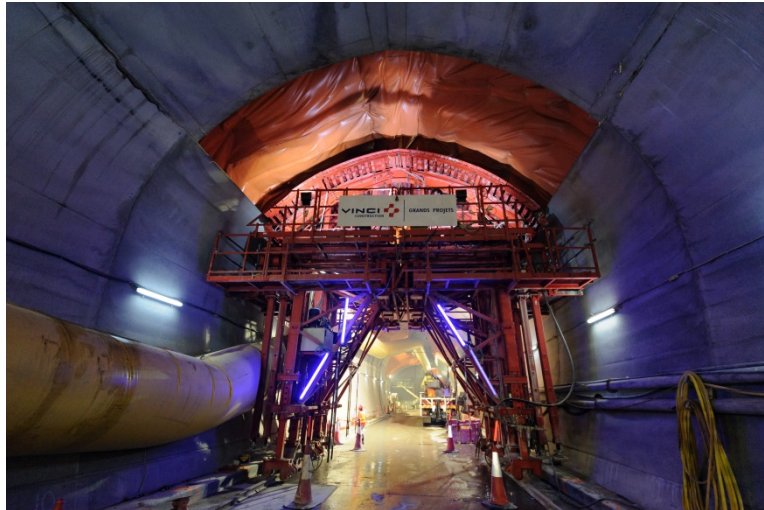
Structural works are being carried out inside the overrun tunnel
