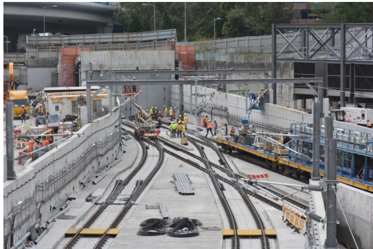
Installation of overhead lines substantially completed at Hung Hom stabling sidings
