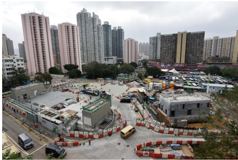
Emergency Access Point at Fung Tak
