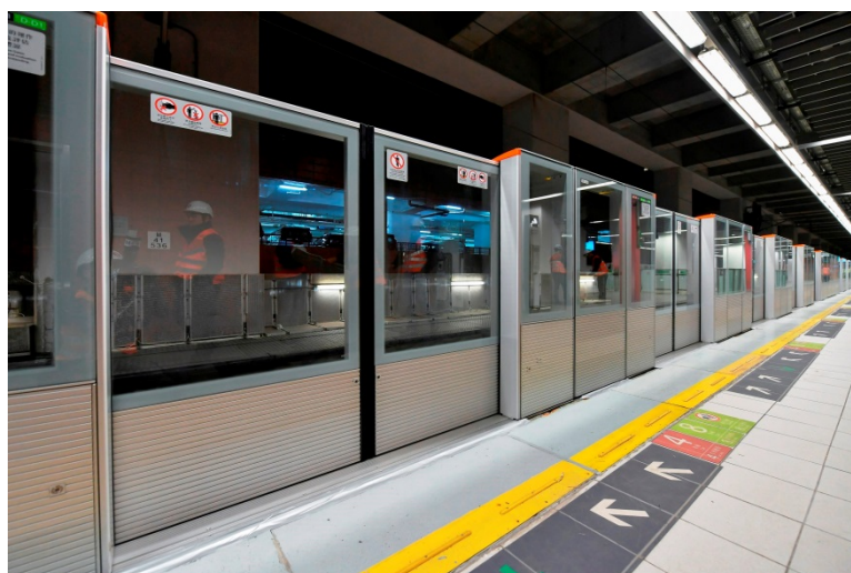
Retrofitting works of APGs at MOL stations completed
