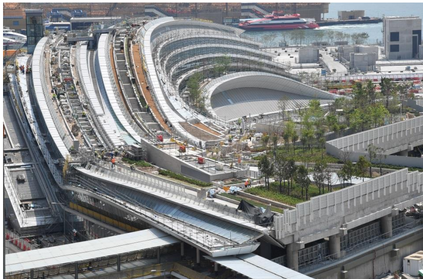
Landscaping works at Hong Kong West Kowloon Station
