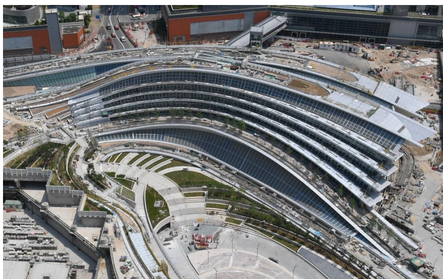
The construction of Hong Kong West Kowloon Station has been substantially completed
