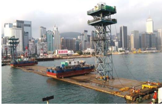
All 11 IMT pre-cast units have been successfully installed in Victoria Harbour
