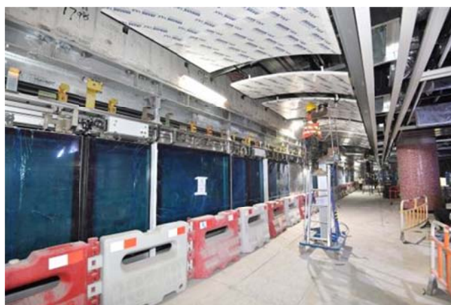
E&M installation in progress at Hung Hom Station
