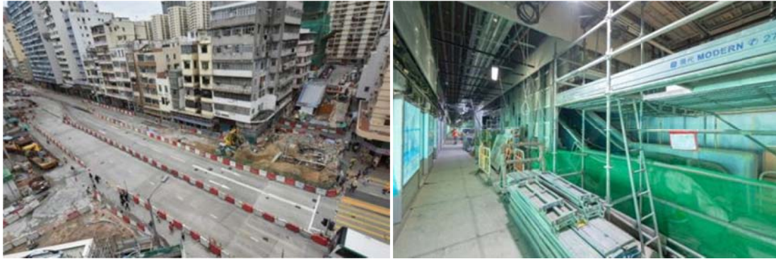
Construction works of To Kwa Wan Station
