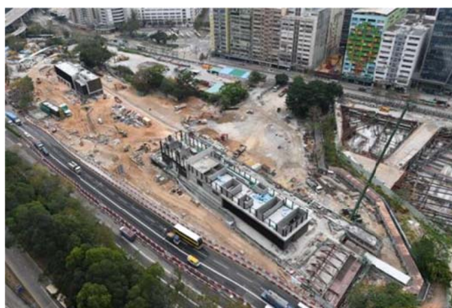
Expansion works for Diamond Hill Station
