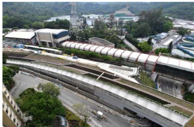
Viaduct and at-grade tunnel box
