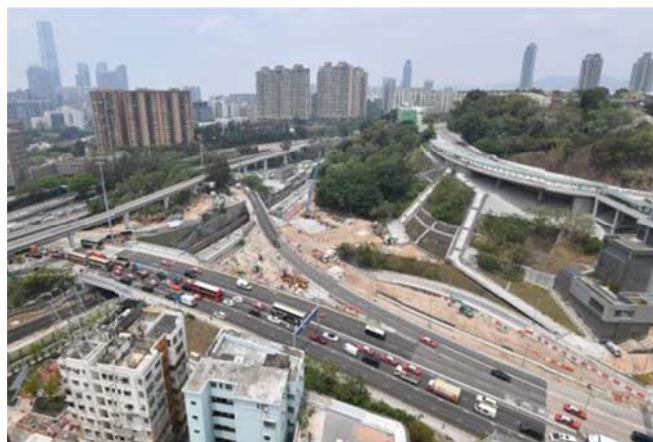
Temporary Traffic Management Schemes completed along Chatham Road North, Winslow Street underpass slip road and Hong Chong Road slip road
