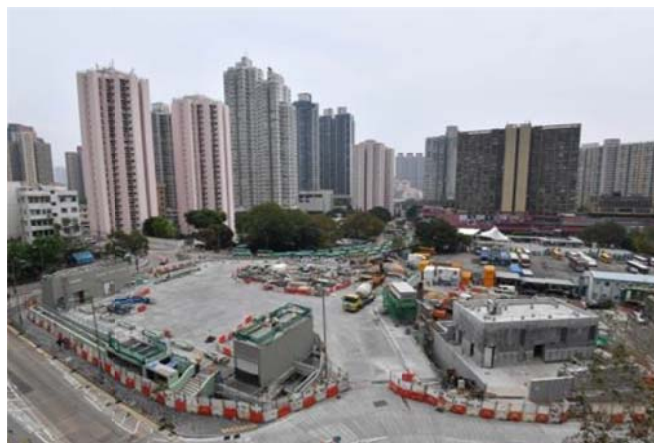
Emergency Access Point at Fung Tak
