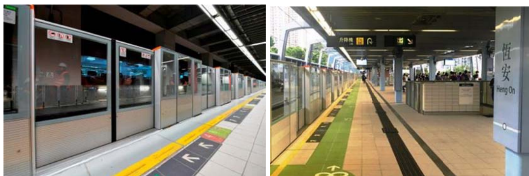
Retrofitting works of APGs at MOL stations completed
