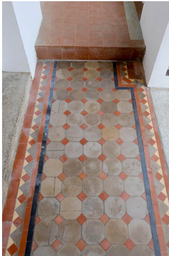
Historic patterned floor tiles at the verandah in the north elevation
