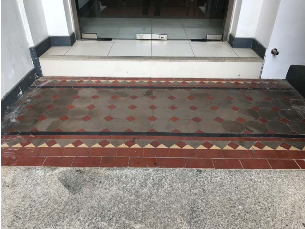
Historic patterned floor tiles at the verandah in the north elevation
