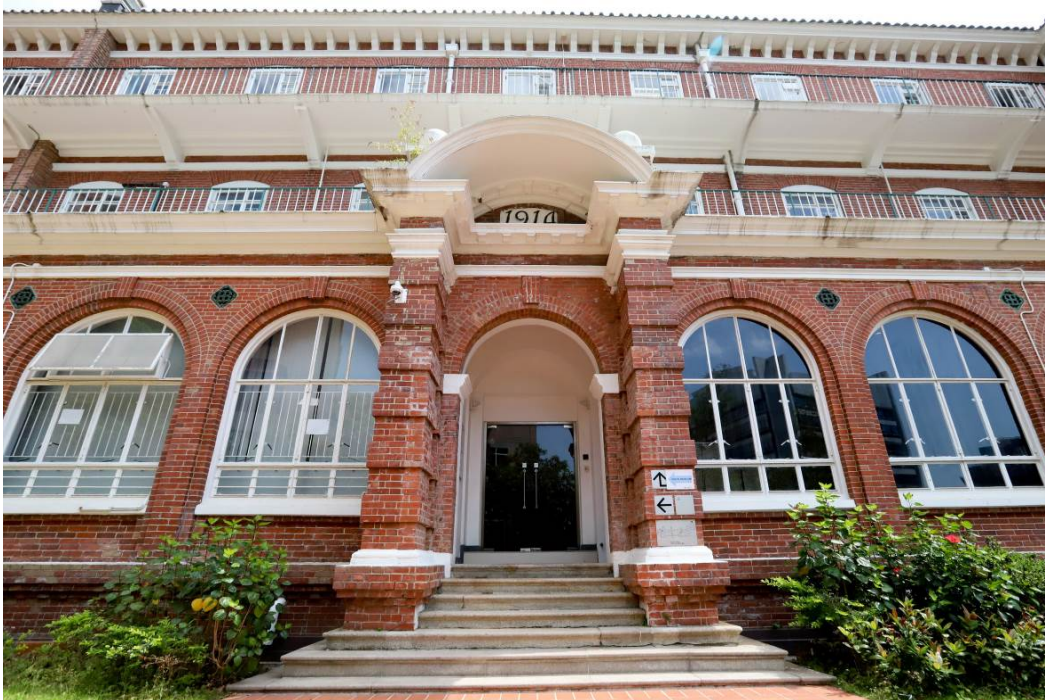
Rusticated brick piers and an elaborate shaped portico at the front facade
