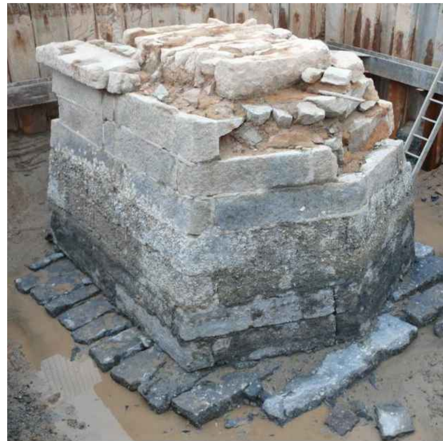
圖B - 橋墩遺跡 (位置見附錄3) FIGURE B - REMNANTS OF STONE SUPPORTING PILLAR (LOCATION OF REMNANTS REFERS TO ENCLOSURE 3)
