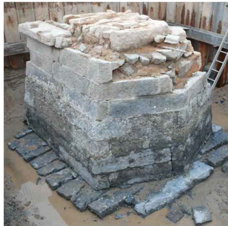
圖B - 橋墩遺跡 (位置見附件3) FIGURE B - REMNANTS OF STONE SUPPORTING PILLAR (LOCATION OF REMNANTS REFERS TO ENCLOSURE 3)
