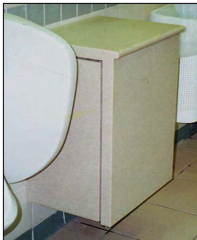
Slop sink in a tailor-made cabinet
