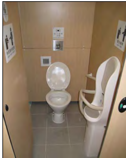
Baby rest (floor standing type with fixed front guard) in pedestal cubicle
