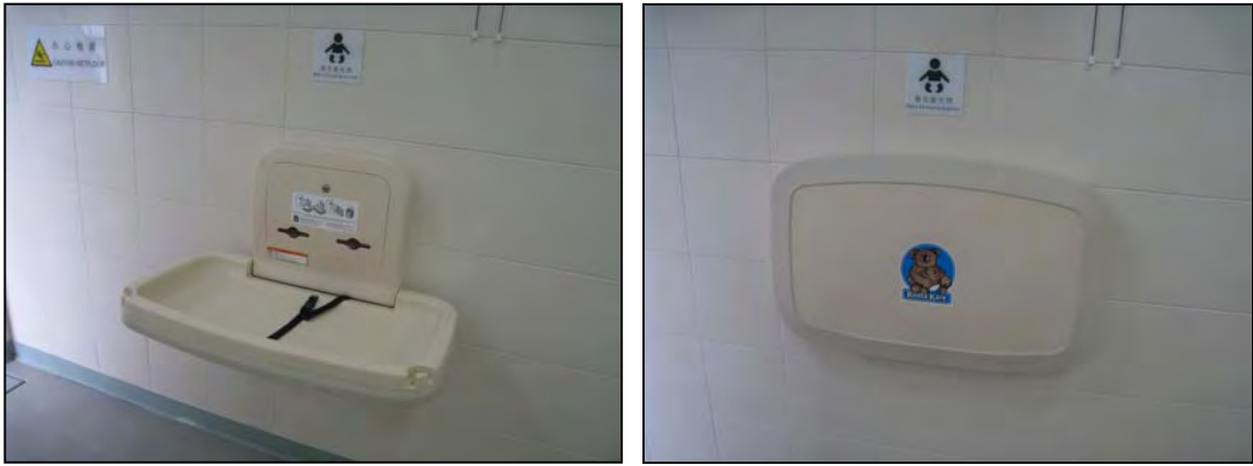
Folding baby changing counter with indicative sign above
