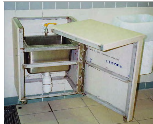
Slop sink in a tailor-made cabinet
