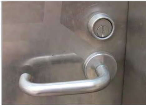
Door lock can be opened with a coin from outside
