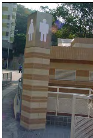
Tai Hang Road Public Toilet (Wanchai)
