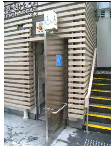
Door swings outward unobstructively
