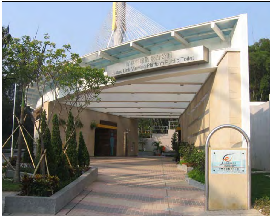
Lantau Link Viewing Platform Public Toilet (Kwai Tsing)
