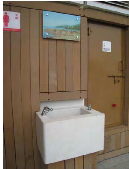
Wash hand trough outside the toilet premises
