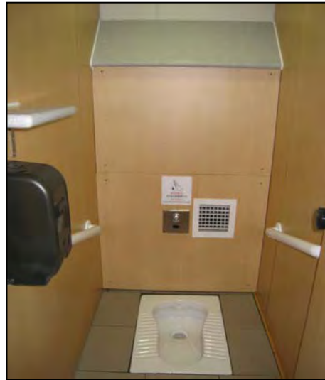
Slanted ledge covering water cistern
