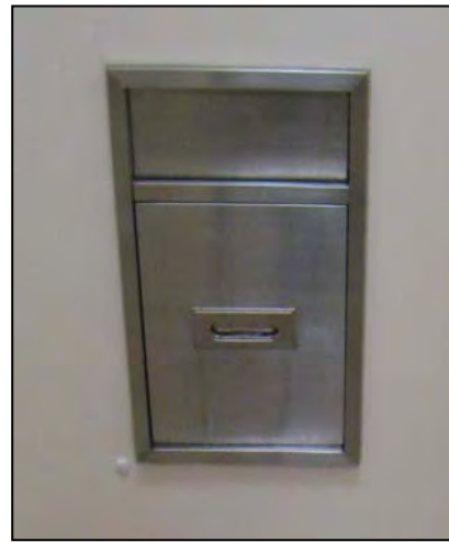
Recess-type sanitary disposal bin
