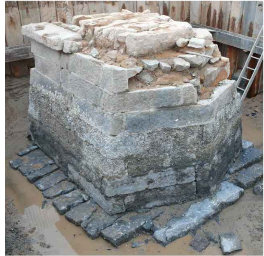
圖B - 橋墩遺跡 (位置見附錄3) FIGURE B - REMNANTS OF STONE SUPPORTING PILLAR (LOCATION OF REMNANTS REFERS TO ENCLOSURE 3)
