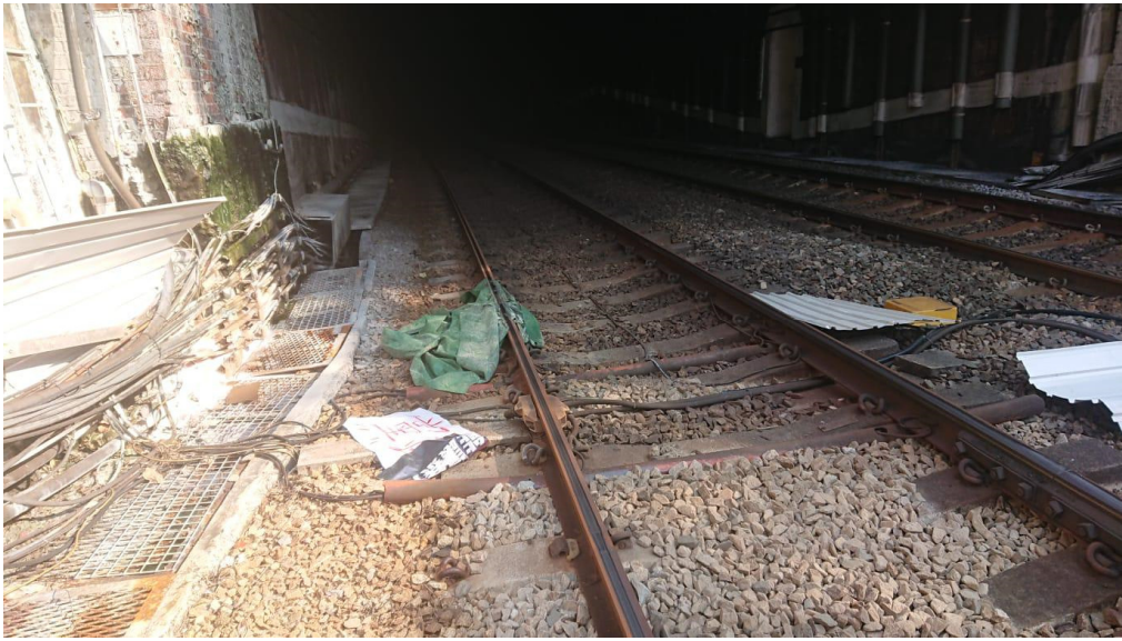
Kowloon Tong Station on East Rail Line
