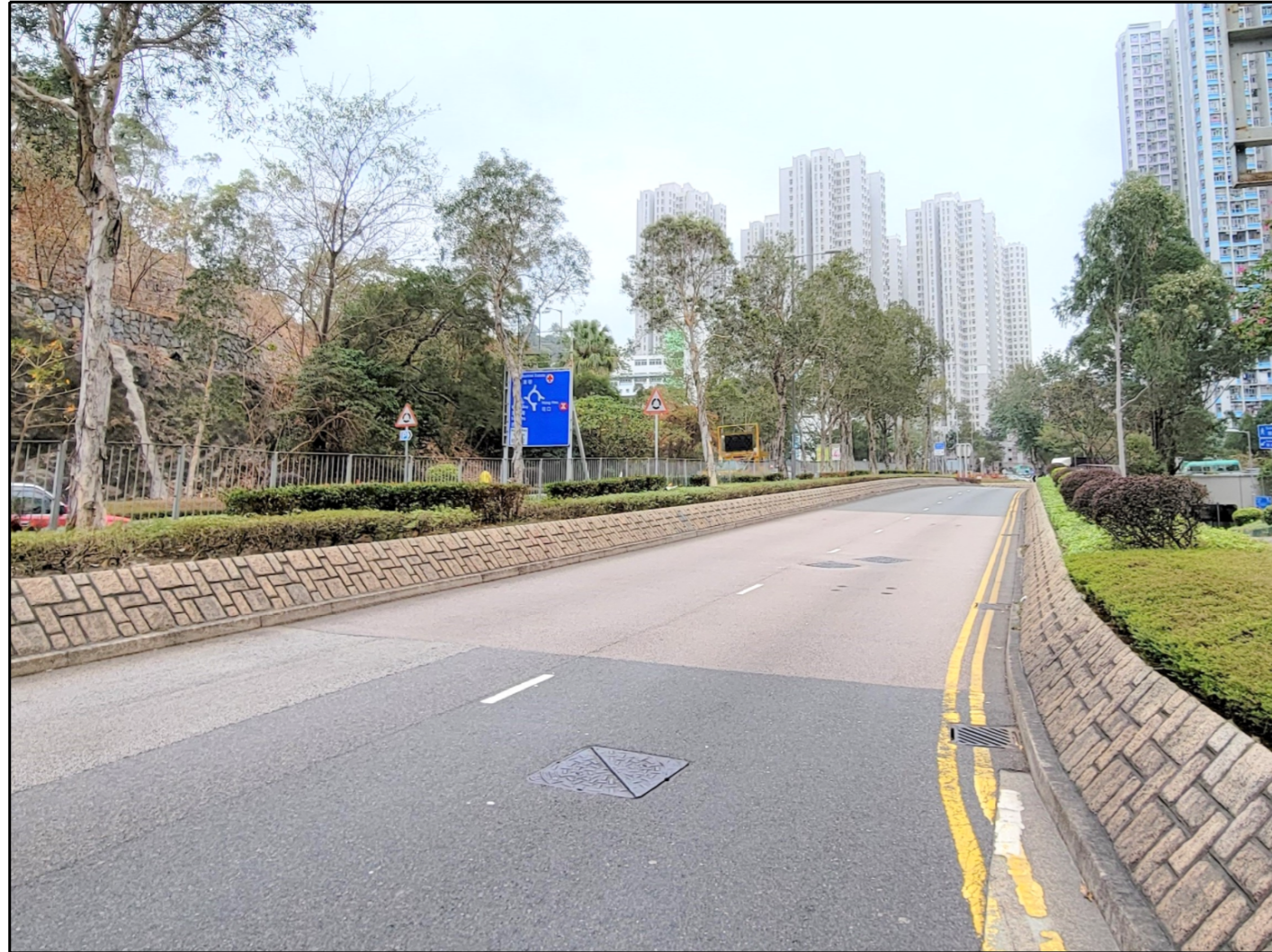
近厚德邨現況 Present Situation Near Hau Tak Estate
