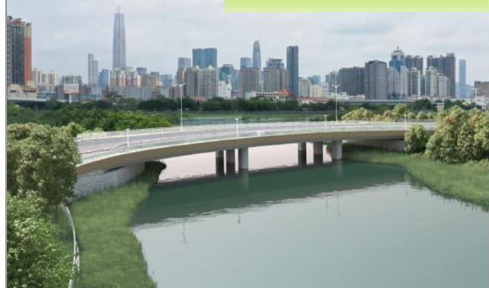
擬議跨越河曲行車橋(包括雙程雙線分隔道路、行人路及單車徑) PROPOSED MEANDER BRIDGE (INCLUDING A DUAL TWO-LANE CARRIAGEWAY, FOOTPATH AND CYCLE TRACK) 視圖A VIEW A
