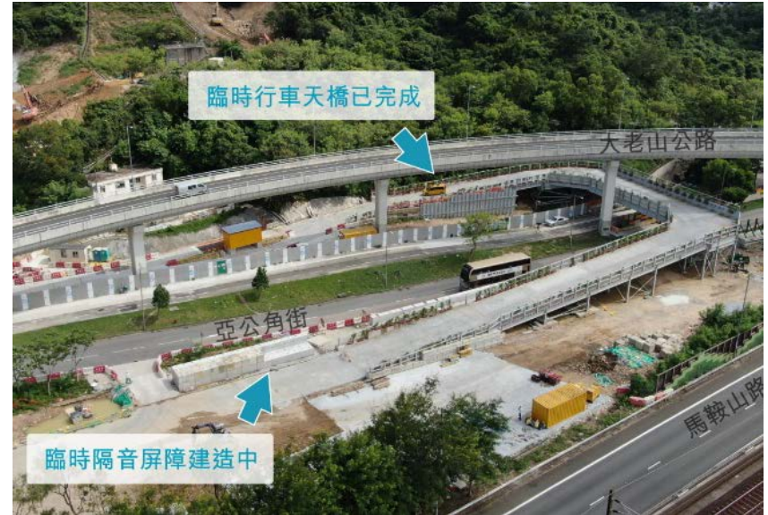
臨時行車天橋已完成 Temporary steel bridge completed
