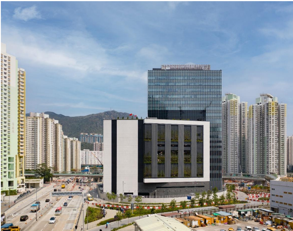
東九龍總區總部及行動基地暨牛頭角分區警署 Kowloon East Regional Headquarters and Operational Base cum Ngau Tau Kok Divisional Police Station
