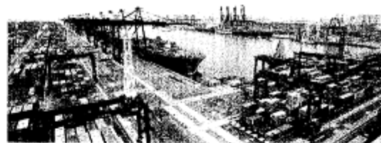
• 葵涌港口設施。 Port facilities at Kwai Chung
