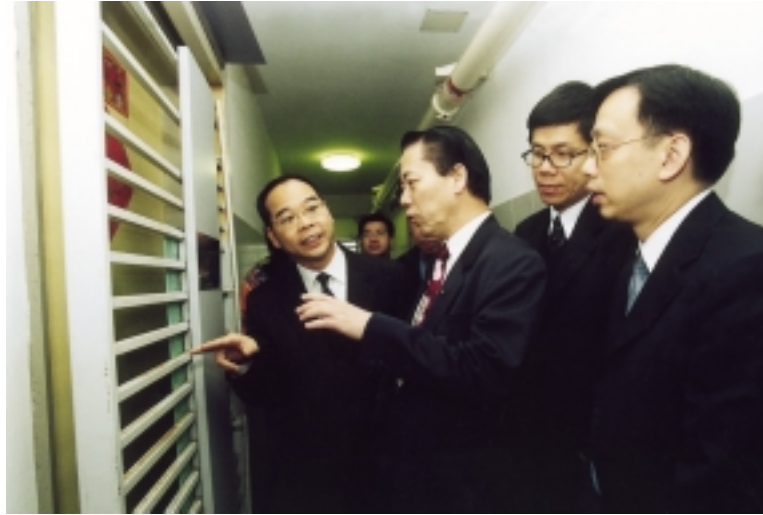
Members on a public housing estate site visit gather information about a complaint concerning rusting gates.
