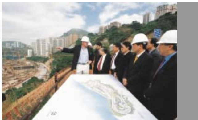
During a site visit, members of the Panel on Information Technology and Broadcasting are briefed by an engineer on the construction progress of the Cyberport project.
