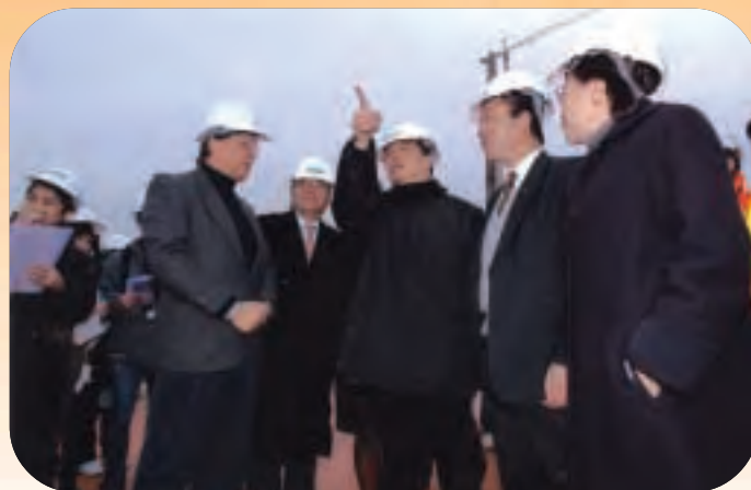
Members of the Panel on Transport visit the site of the Hong Kong-Shenzhen Western Corridor landing point in Ngau Hom Shek to be briefed on the progress of the project.
