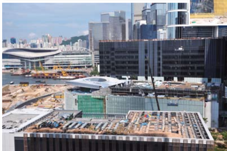
Construction work of the Legislative Council Complex in progress.
