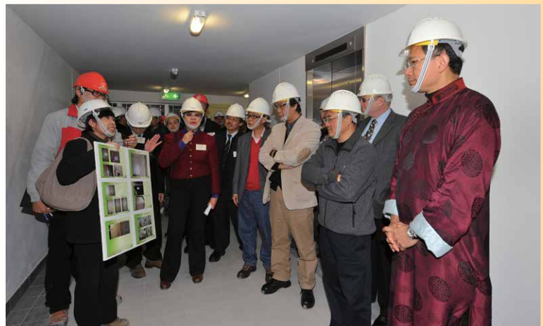
Members of the Panel on Housing receive a briefing on the “Homes in the Park” theme adopted for the design and construction of housing projects during a site visit to a public housing construction site in Kai Tak.
