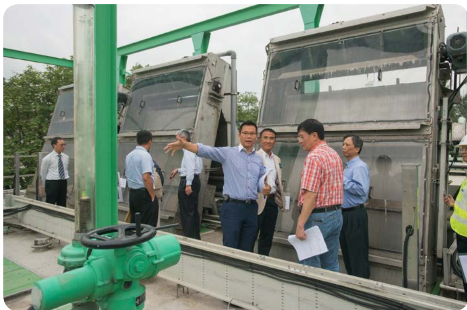
Members of the Panel on Environmental Affairs inspect the treatment facilities of the Pillar Point Sewage Treatment Works in Tuen Mun.
