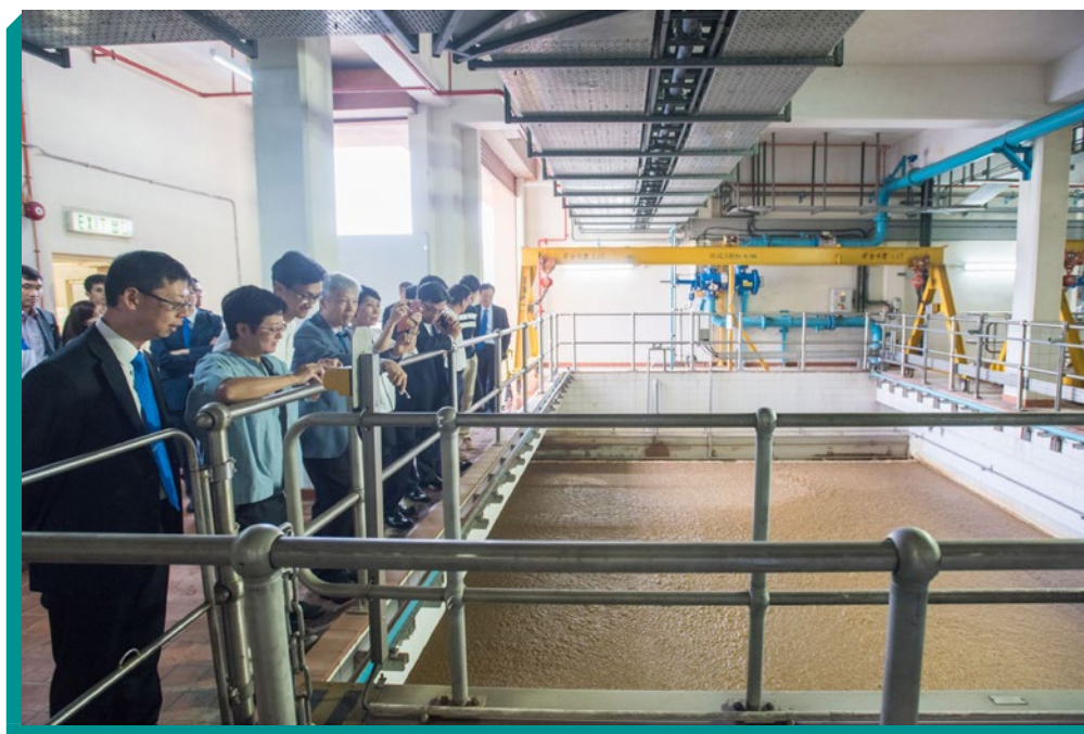
Panel members visit the Dissolved Air Flotation Plant at Tai Po Water Treatment Works to observe the operation of the Dissolved Air Flotation Clarifier.
