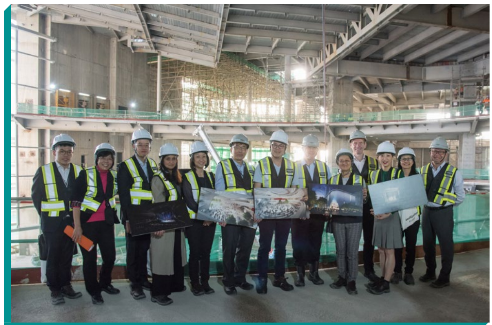
Joint Subcommittee members visit the construction site of the Xiqu Centre, the first major performing arts venue in WKCD.
