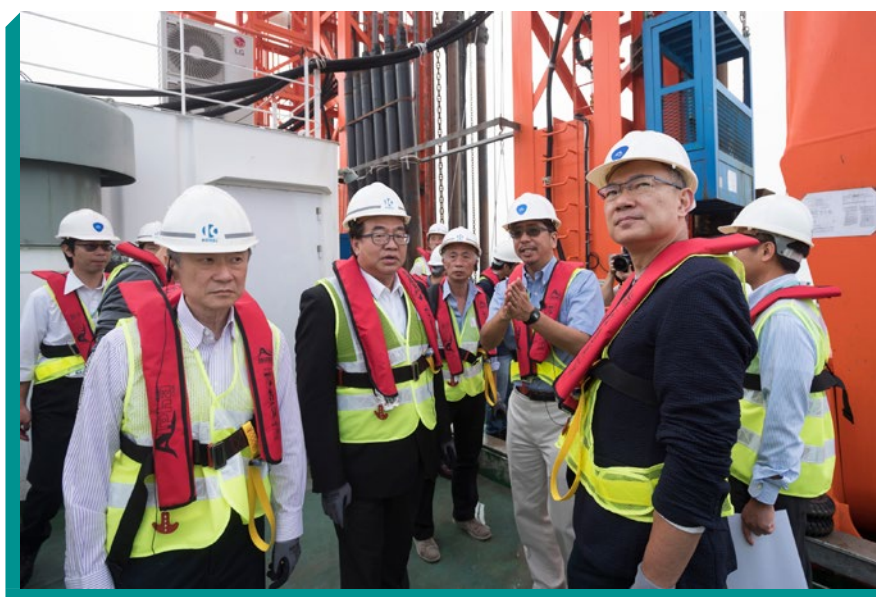
Subcommittee members observe from a close distance how deep cement mixing method was used for non-dredge reclamation.
