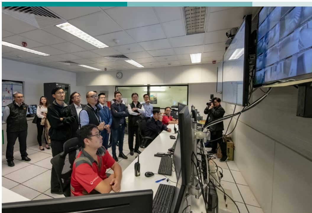
Members of the Public Works Subcommittee tour the control room of North District Cooling System Plant at Kai Tak Development.
