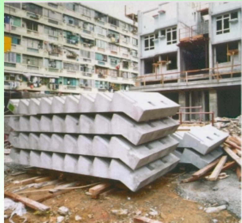
預製樓梯 Prefabricated stair flights
