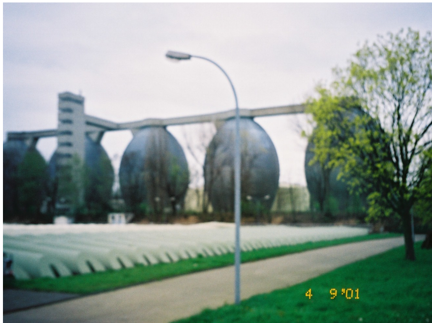
Sludge digestors
