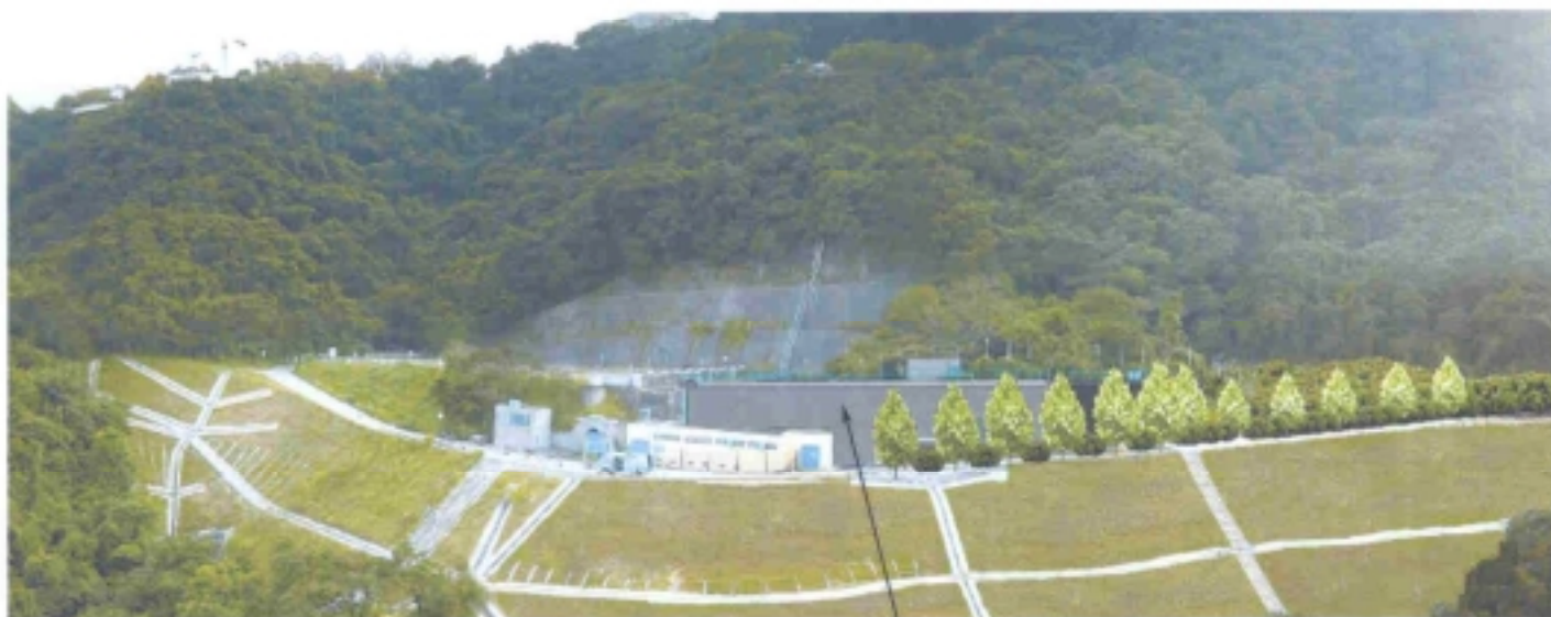
擬建的馬己仙峽道三號食水配水庫 配水庫：49.6米(長) x 22.6米(闊) x 6.1米(高) PROPOSED MAGAZINE GAP ROAD NO. 3 FRESH WATER SERVICE RESERVOIR SERVICE RESERVOIR : 49.6m( L) x 22.6m(W) x 6.1m(H)
