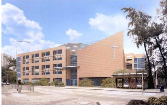
電腦繪製的新校舍模擬圖(南面) Computer rendering drawing of the new school building (Southern View)
