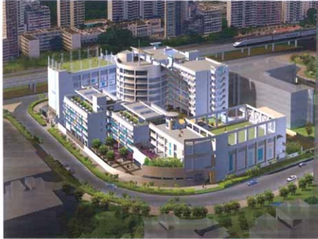
電腦繪製的工地概觀圖(西北面) COMPUTER RENDERING DRAWING OF THE SITE (NORTH-WESTERN VIEW)
