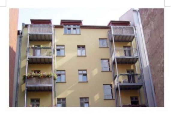
Photo 4.3 Refurbished residential block (with addition of balconies) at Prenzlauer Berg
