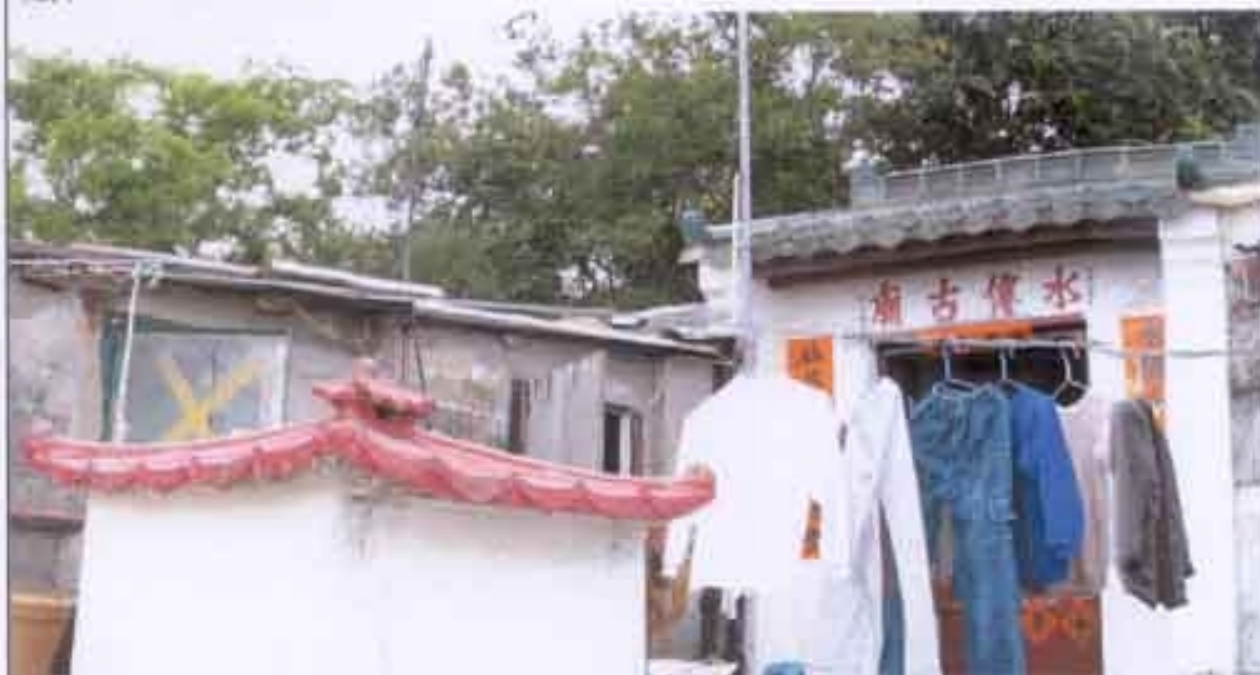
现状 EXISTING CONDITION
