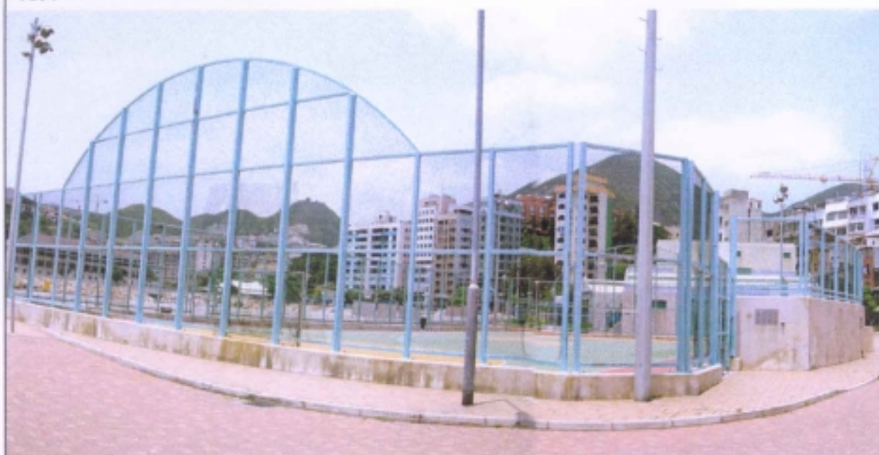
現狀 EXISTING CONDITION
