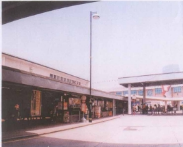
現狀existing condition
