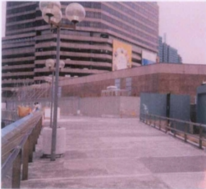
現狀existing condition
