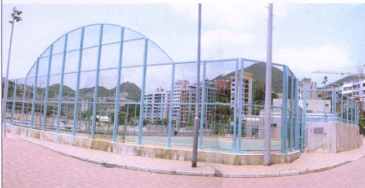
現狀 EXISTING CONDITION
