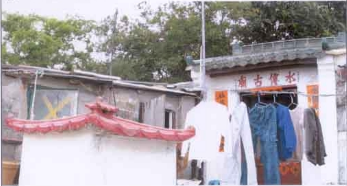
現狀 EXISTING CONDITION
