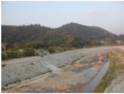
Ng Tung River, Fanling, after Channelization works
