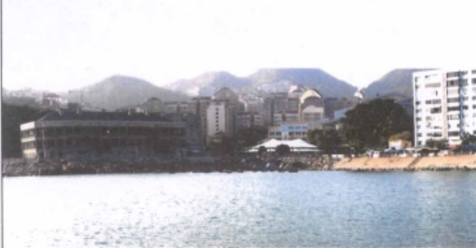
現狀 EXISTING CONDITION
