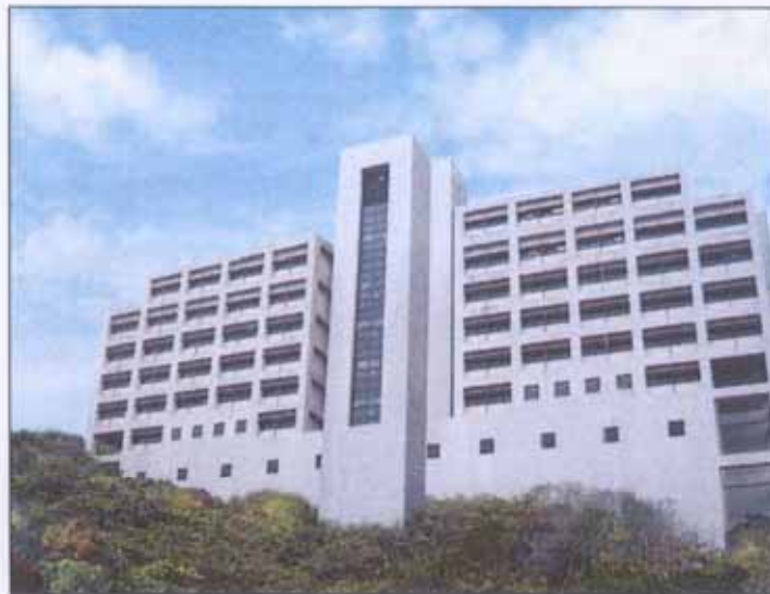
專科門診大樓南面立面圖 (模擬圖 - 改善工程後) South Elevation of the Specialist Outpatient Block (Artist's Impression - After Improvement)
