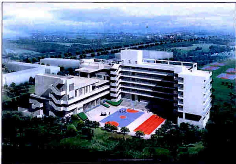
VIEW OF THE SCHOOL PREMISES FROM SOUTHEAST DIRECTION (ARTIST'S IMPRESSION) 從東南面望向校舍的構思圖
