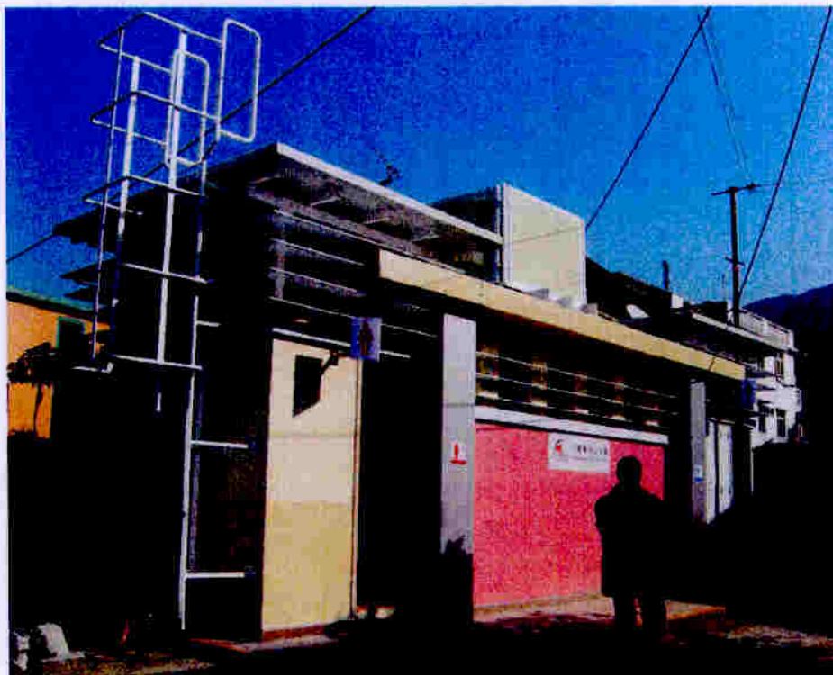
廁所改善後之外貌 EXTERIOR VIEW OF TOILET AFTER IMPROVEMENT
