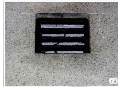
Photo P26 – Opening for Ventilation in Snack Shop/Store Room 相片 P26 – 小食店/士多層的氣窗
