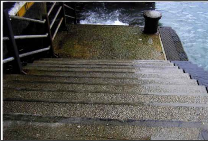
登岸階梯的預製混凝土條及扶手 Precast concrete landing steps and handrails
