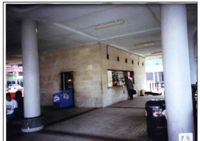
受力牆的石面 The stone facing of the load bearing wall
