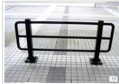
Photo P8 - General View of Railing in the Edge of Pier 相片 P8 - 碼頭外圍的欄杆
