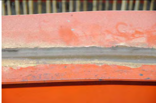
Fig. 4: Rust and peeling coat of paint at the coupling rails
