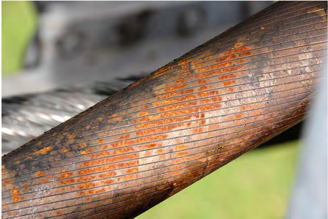
Figure 18 – Close up view on the track rope with rust
