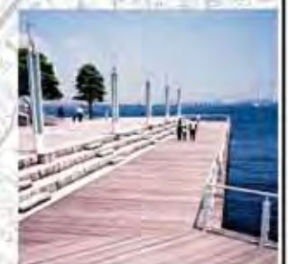
19. Boardwalks will be used to create an interesting edge to the typhoon shelter and marine basin
