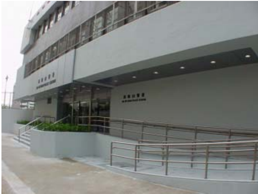
Improved Station Entrance
