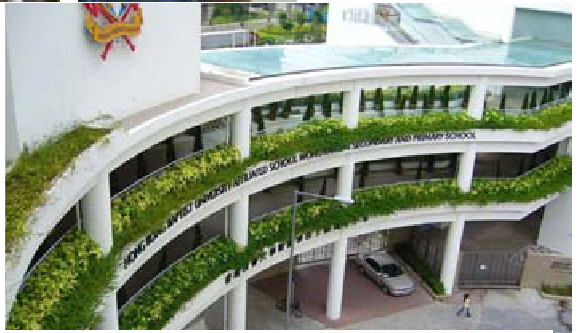
Roof and podium garden at a Secondary-cum Primary School in Area 11, Sha Tin 在沙田第11區一所中學暨小學的屋頂及平台花園
