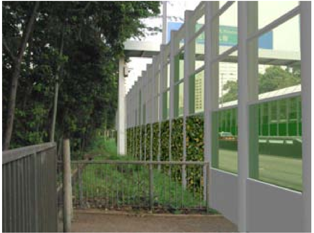
Green noise barrier on Tsing Tsuen Road near Riviera Gardens 青荃路近海濱花園的綠化隔音屏障
