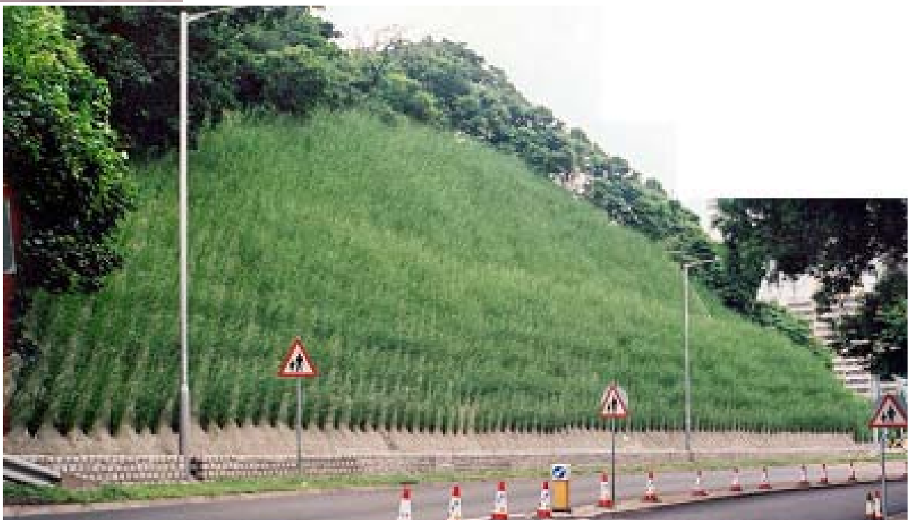
Slope at Lion Rock Tunnel Road 獅子山隧道公路的斜坡
