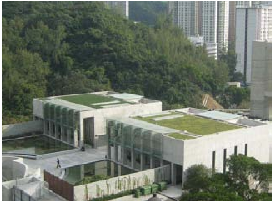
Green roof and vertical greening at Diamond Hill Crematorium 鑽石山火葬場的屋頂綠化及垂直綠化
